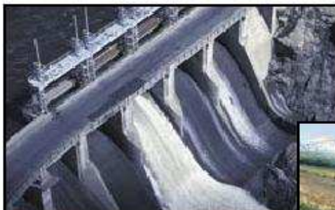
Flood Gate Control/Irrigation
